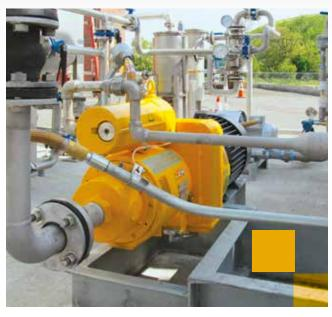
Mattei GC 111 Gas Compressor and 50 HP motor to compress Methane gas to drive a Capstone Micro Turbine to generate electricity used at the site.
