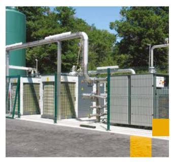
Installation of 5 Mattei 55 kW gas variable speed compressors with a pressure of 8 bar which can compress up to 9,000 litre a minute of biogas containing up to 300 ppm of hydrogen sulphide, in accordance with the microturbine specifications.
